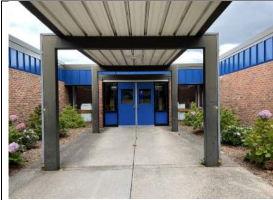
Image 1 – Exterior view of main entrance and entrance door illustration blue cladding placed over limestone elements.
