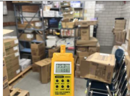
Image 20 – Overall interior view of Gymnasium. Relative humidity in the Boy’s Locker Room space was observed to be approximately 35% prior to pressurization.
