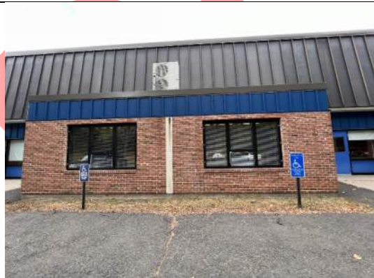
Image 15 – Partial south elevation view of Room N. New windows have been added since the original construction drawings did not indicate windows at these locations.
