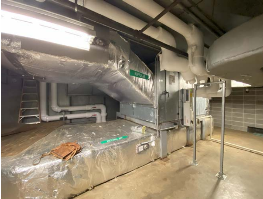
Existing Cafeteria unit Where heat pipe will be installed
