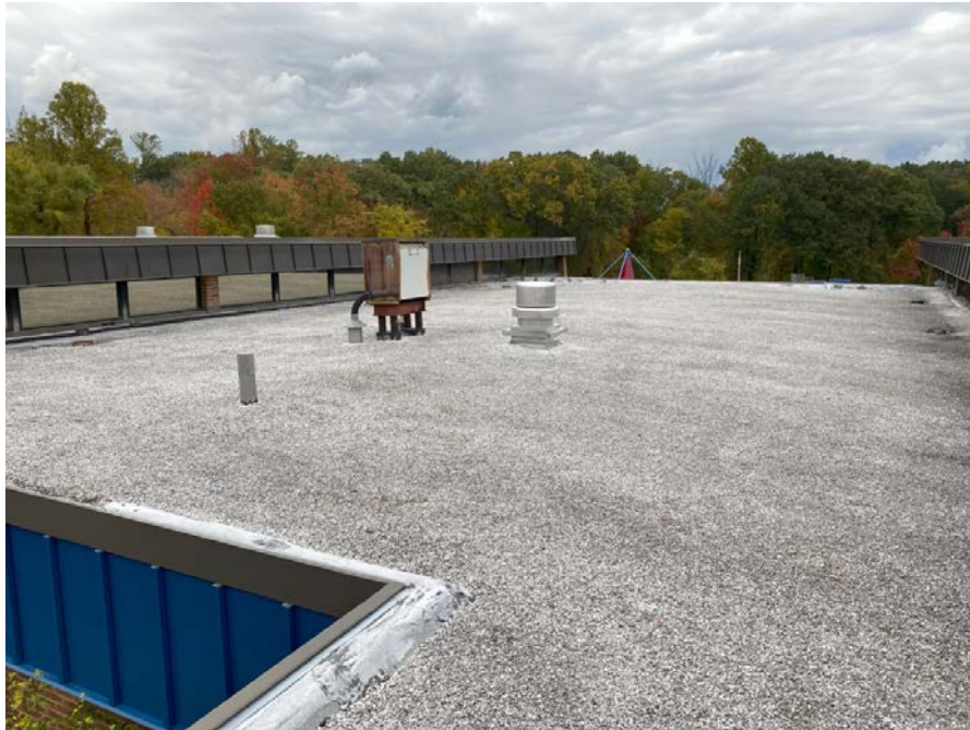
Lower roof where new DOA units will be placed
