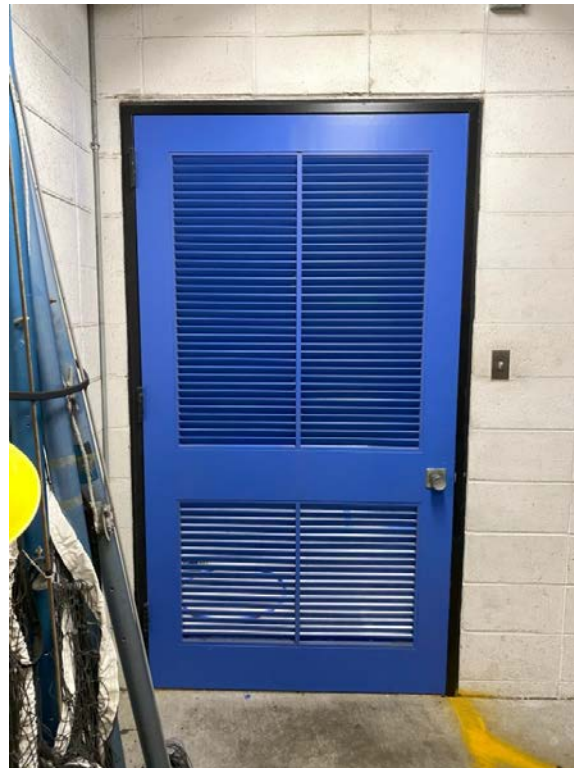
Louvered door in Gym storage room
