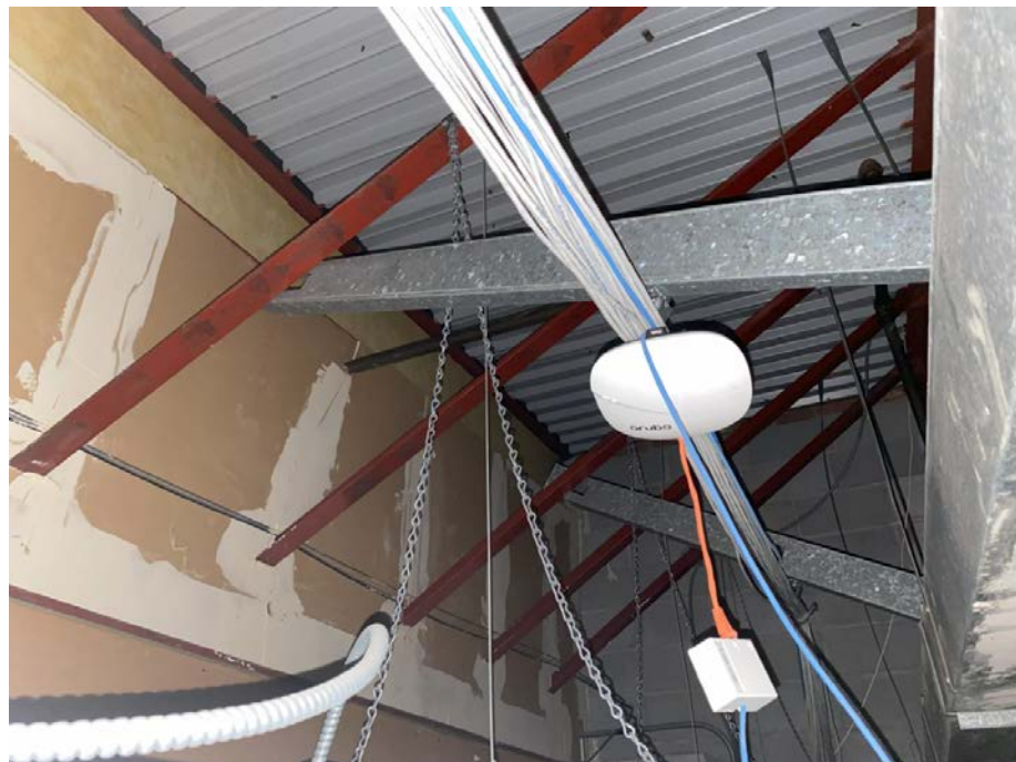
Ceiling cavity where new ductwork from DOAS units will be run
