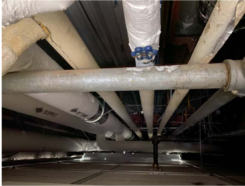
Ceiling space in Corridor area
