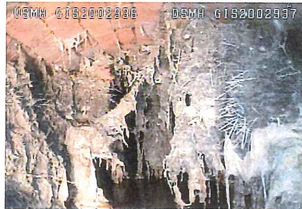
Old North Branch Interceptor Hartford
