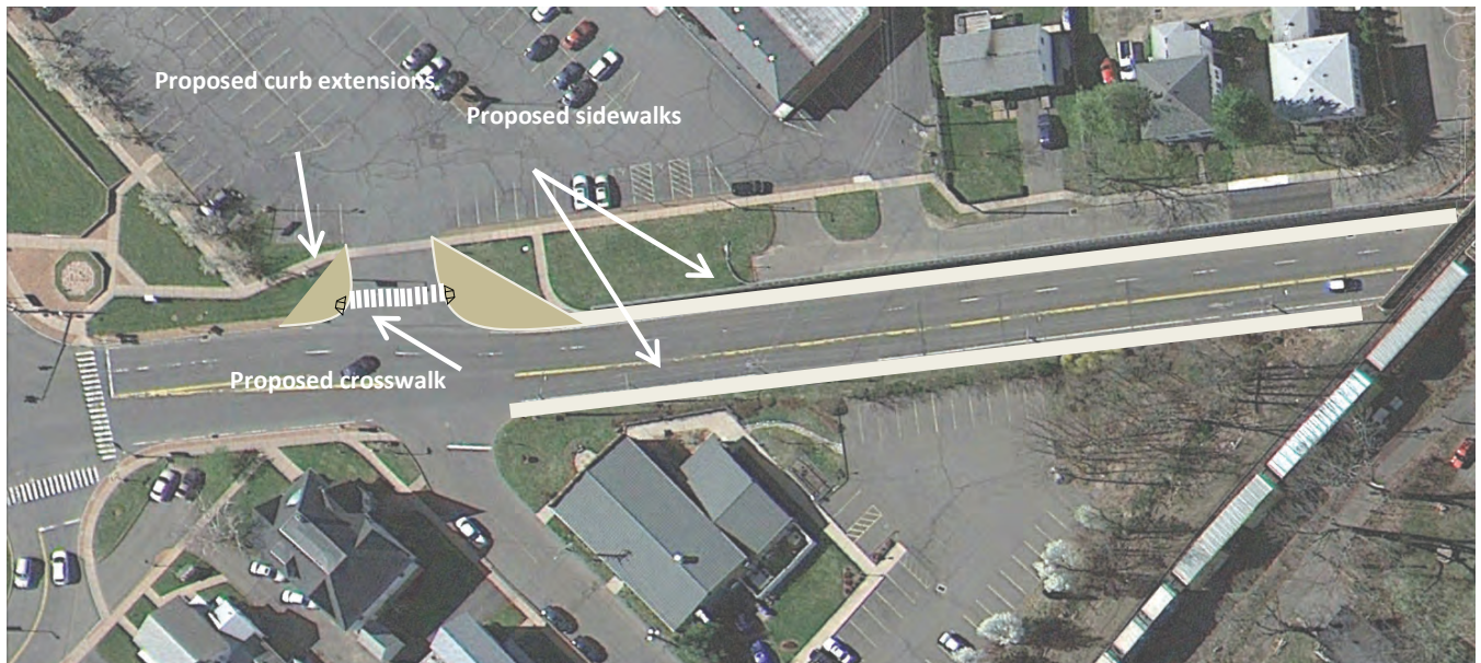
Figure 18. Pedestrian Facilities on Palisado Avenue
