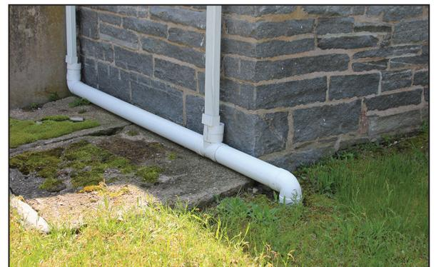
Figure 1. Gutter downspout connected to underground pipe.
