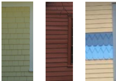
Wood Shingle Horizontal Clapboard Unique Original Shingles
