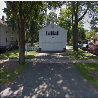
Inappropriate Raised Ranch
