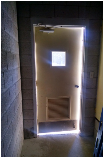
Current Entry / Exit Door to Bathrooms
